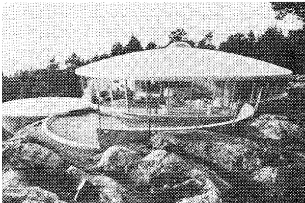
Figure 8: House with plastic construction, Staffan Berglund, Torö, in the archipelago of Stockholm, 1970. (Picture from, "Handboken Bygg, Material...", Stockholm, 1984, p. 306.)
